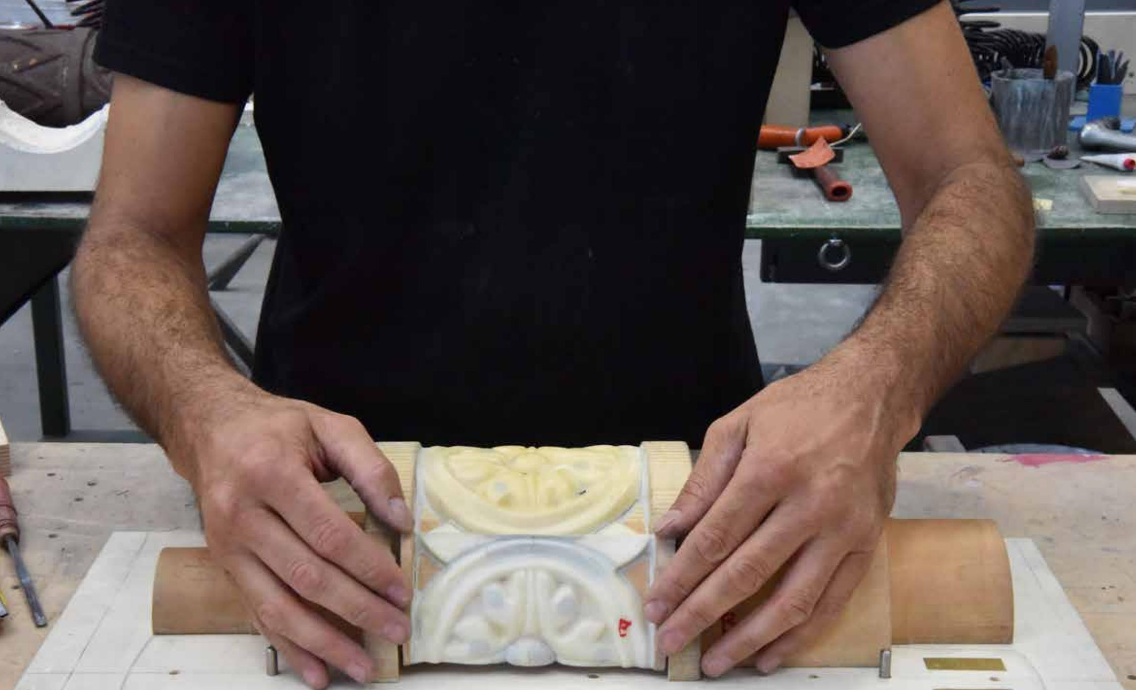
Once the new castings had been lathed and inserted in the columns, a perfect joint between the two parts was obtained.
