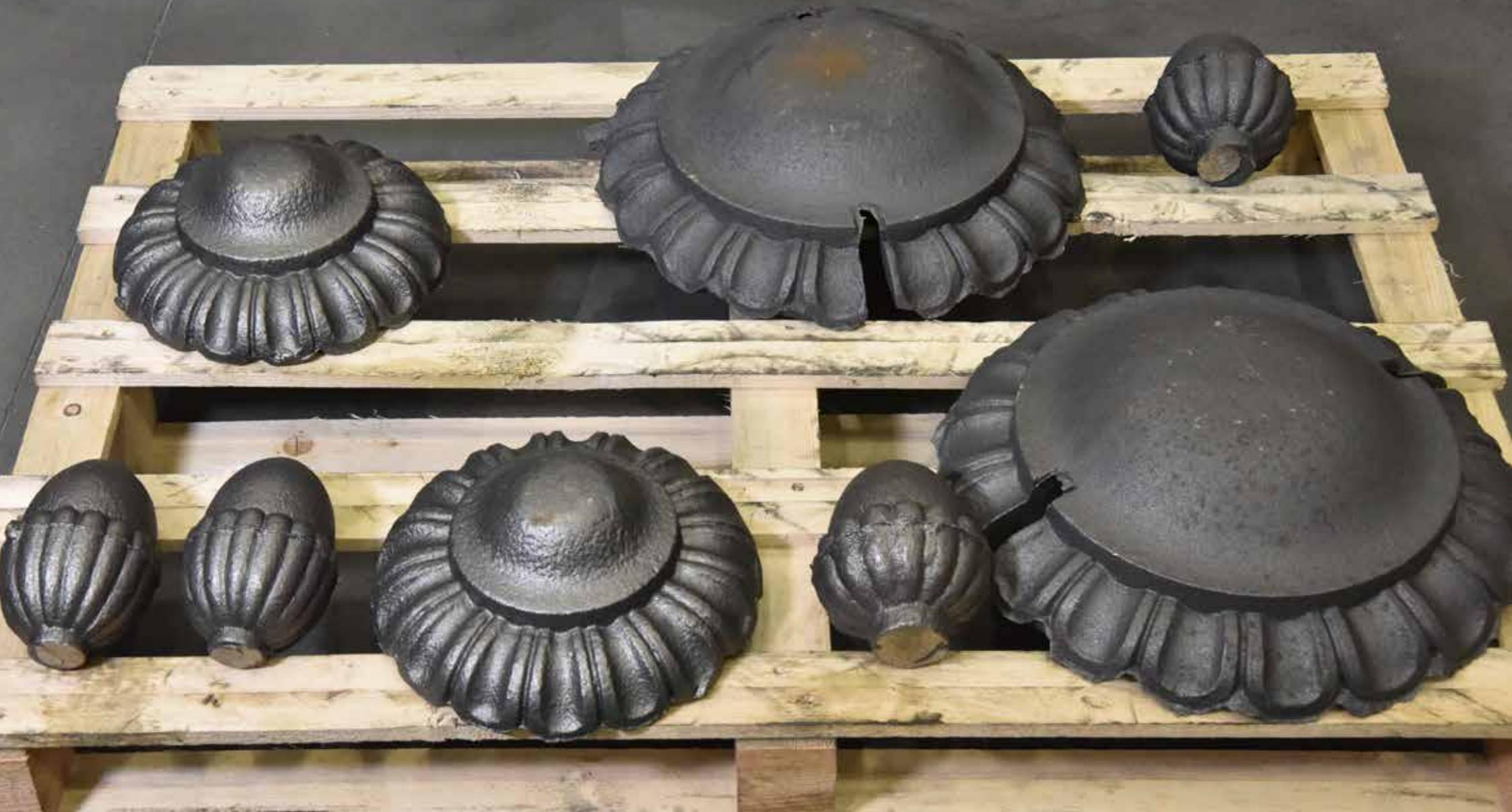
The 23 arches of the pergola were originally linked by a decorative upper strip – to all effects lacework in cast iron – which connected the columns. A census was made of all the items and they were evaluated on the basis of their state of conservation. Incomplete parts capable of retrieval were welded and restored to their original form and dimensions. Missing parts were supplied by castings from new models.
