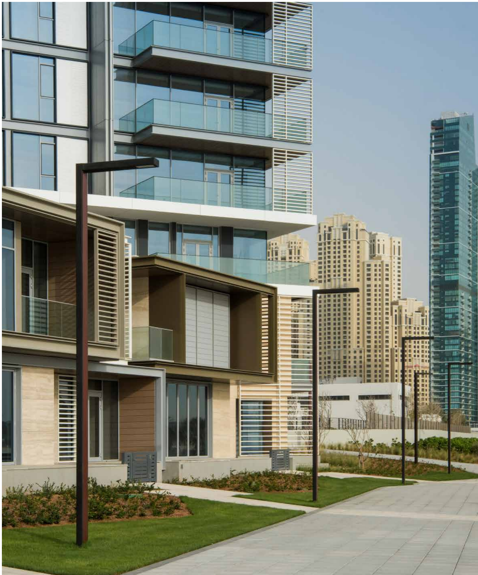
Pictor lighting system h 5 m
