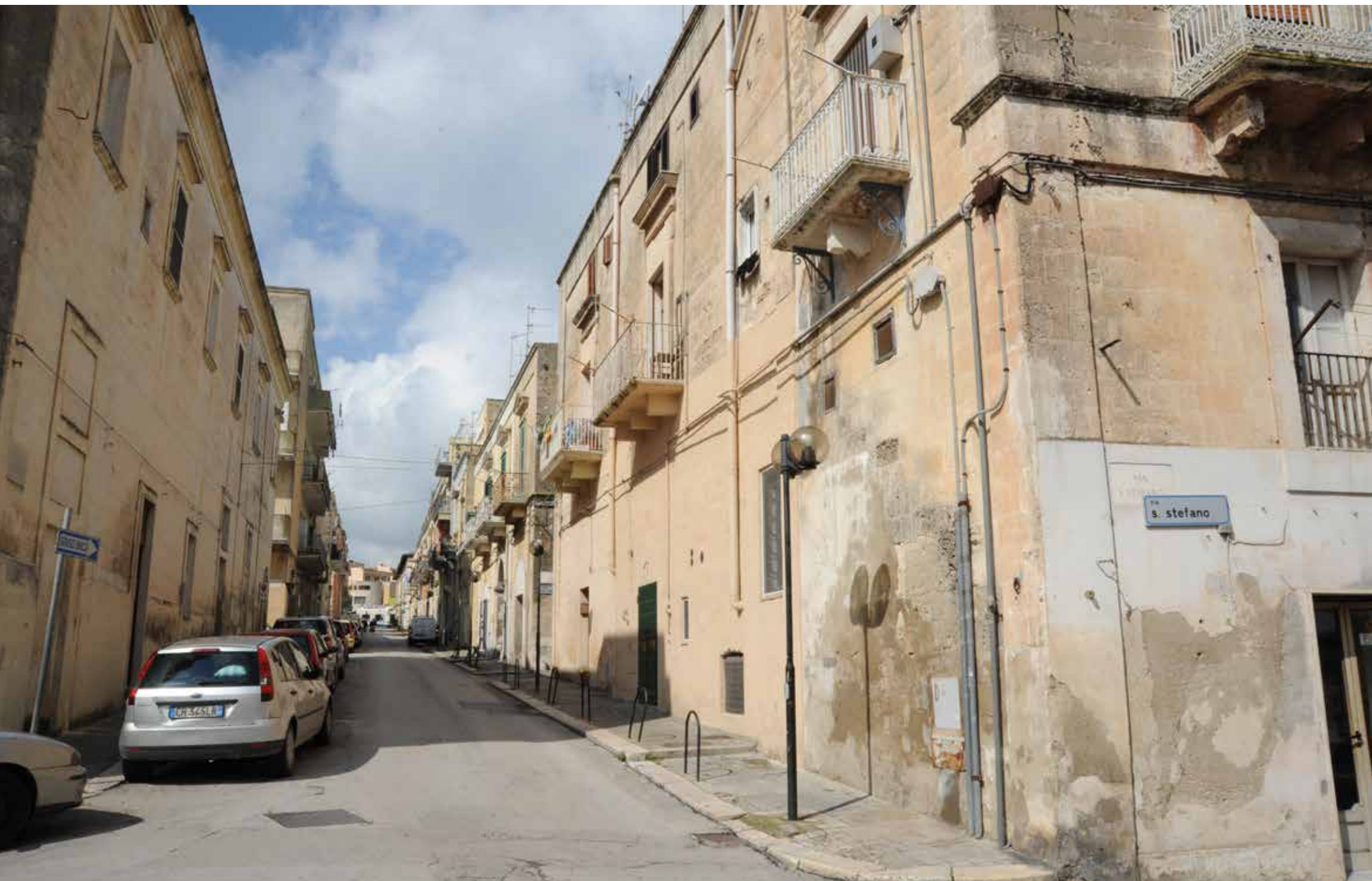
Via Piave with the old lamp posts
